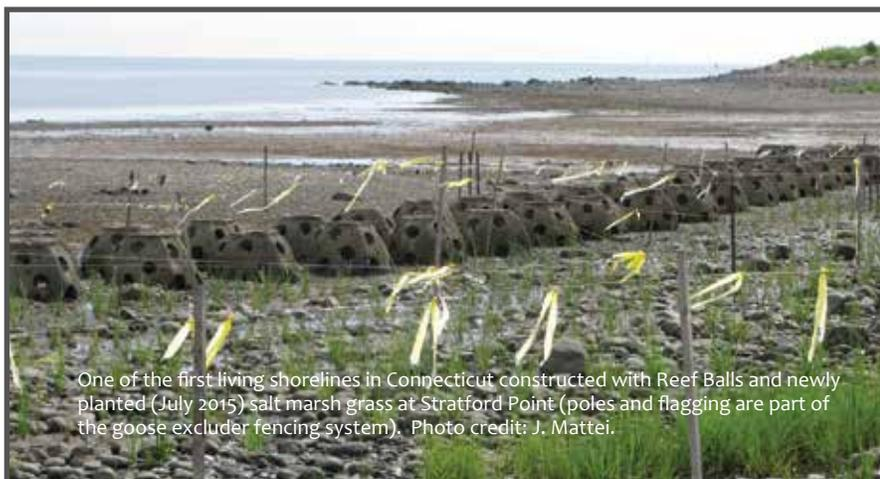
One of the first living shorelines in Connecticut constructed with Reef Balls and newly planted (July 2015) salt marsh grass at Stratford Point (poles and flagging are part of the goose excluder fencing system). Photo credit: J. Mattei.
